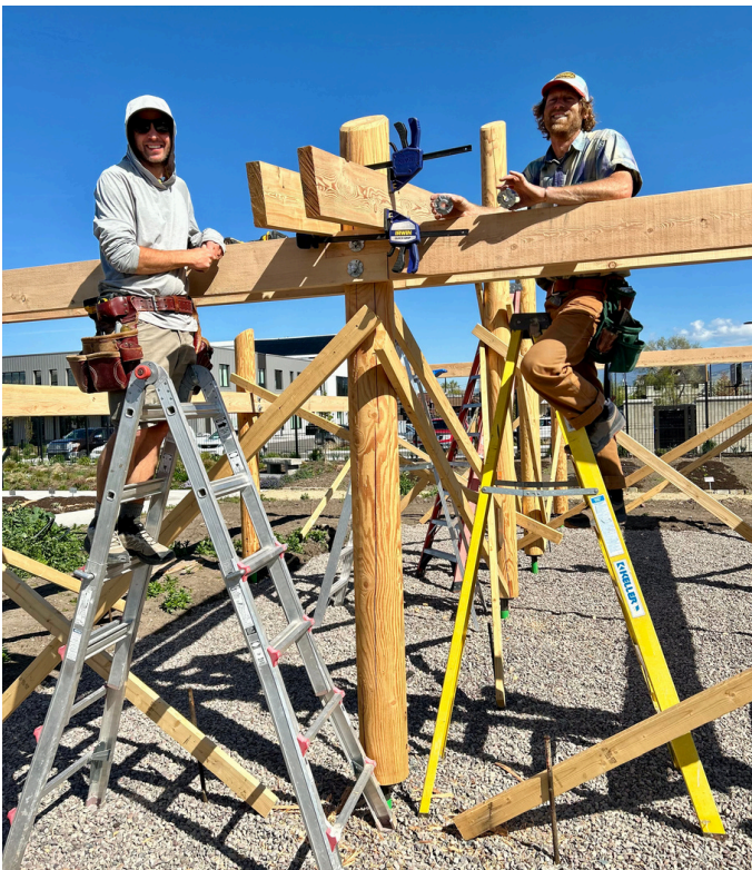
Brandon Zook (left) and David Boden (right) assemble the hardy kiwi arbor, a timber frame structure designed by David, owner of Chisel & Mallet Woodworking.
